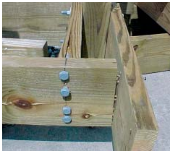
Figure 3. After testing the bolted and lagged connections, the authors tried reinforcing the post with blocking in a variety of configurations. Each configuration they tried failed when the blocking split along the grain.
